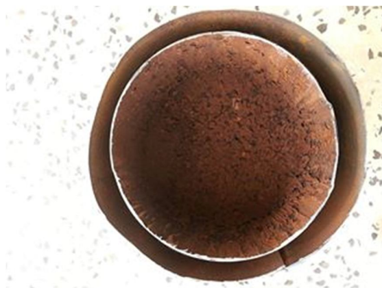
Figure 1. Horizontal cross-section of metallic boiler showing the environmental effects
